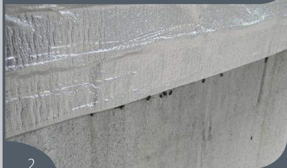
Aluminum faced tape used as a barrier for darkling beetles
