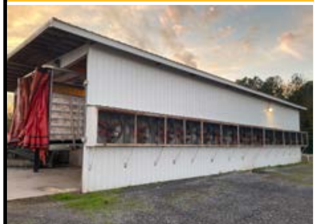
Figure 4.6 Example of appropriate holding facilities at the processing plant.
