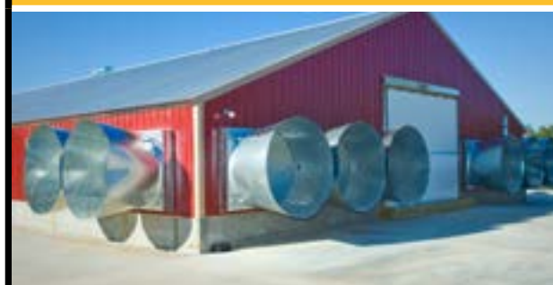
Figure 6.17 Example of a typical tunnel-ventilated house.
