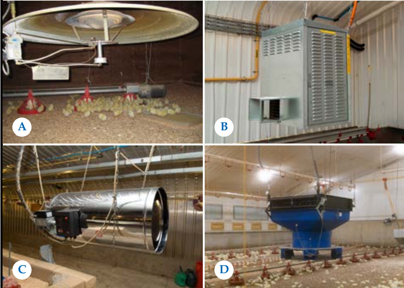
Figure 6.3 Examples of different house heating systems: canopy brooder (A), box heater (B), space heater (C) and hot water air heater (D).
